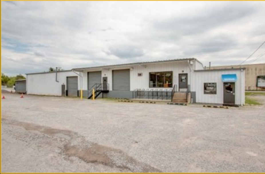
Building exterior, drive-in doors and yard
